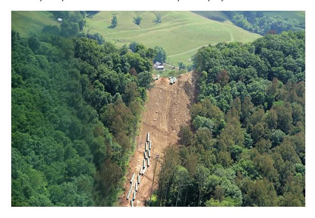
Stonewall Gathering Pipeline Construction in Rugged Mountainous Terrain – Up One Side, Across the Top and DOWN the Other Side.
